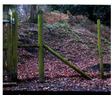
Solid bracing like this is required on strainer posts, near gates and along particularly long fencing runs where additional strength is needed
